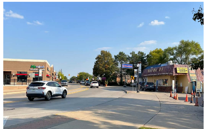
Sidewalks along both sides of the road on Main Street.
