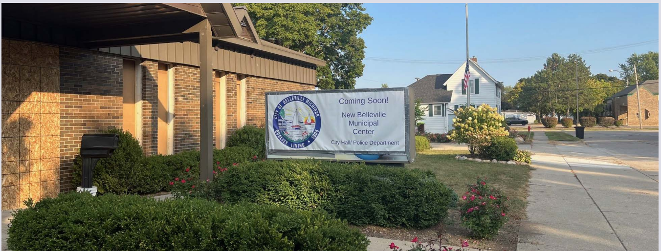
New City Hall location on Charles Street during construction late 2025.
